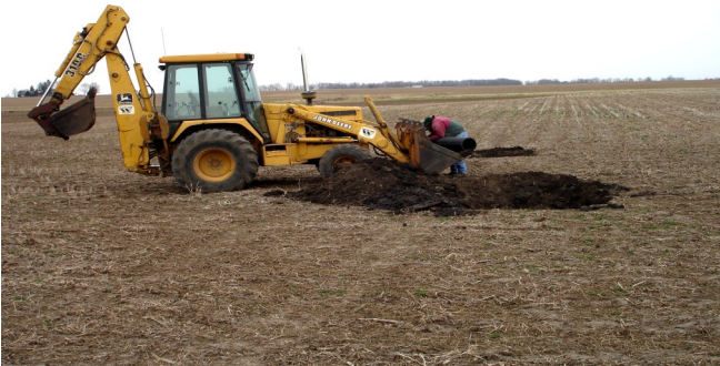
Tim repairing tile
